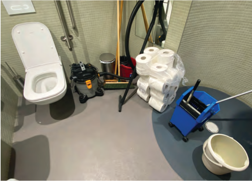
Accessible toilet used as storage. Photo: Jos Boys.
